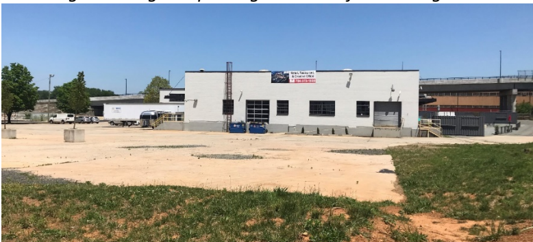
The Bridge building and parking lot – view from the light rail:
